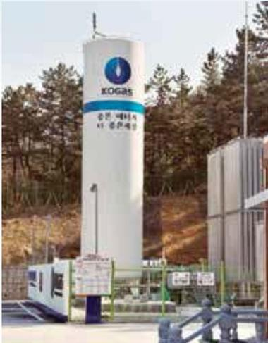
LNG refueling, often used for buses and/or refuse trucks, is more simplistic in design compared to an LCNG station. To transfer LNG from the storage tank to the on-board vehicle tanks for buses and/or trucks, ACD's TC-34 submerged pumps are used.
