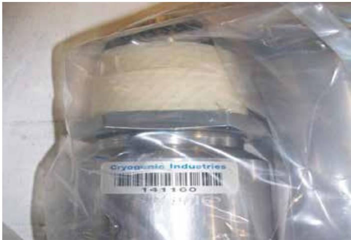
pump with a bar-coded serial number with which to track the pump. The pump's repair history with costs is then recorded for effective equipment management by the customer.
